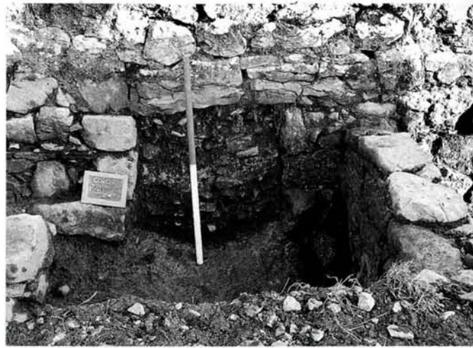
Illus. 6 – Cess egress hole cut into cloister wall. Scale 1m (TVAS [Ireland] Ltd)
