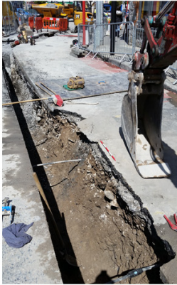
Plate 1: Typical watermain trench. Scale 0.5m
