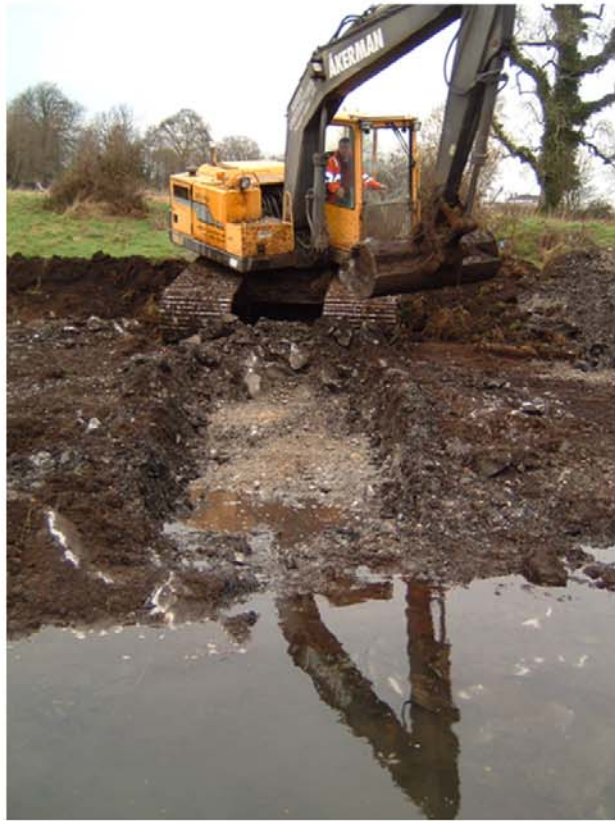
Plate 7. Site AR127 (viii). Looking west
